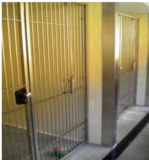
Drainage and building materials
